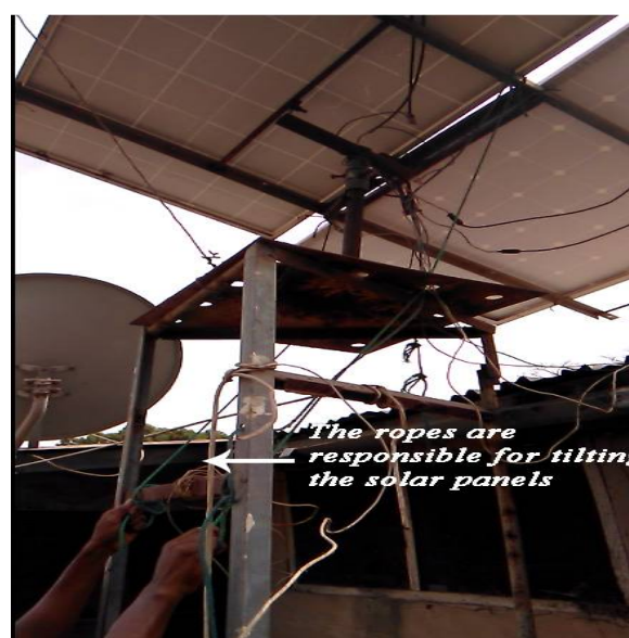
Fig. 4. Manual solar tracker with ropes which need to be manually tilted towards the direction of the sun
